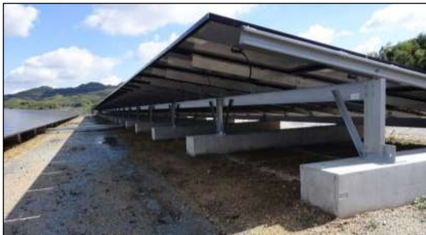
Figure 4: Cast Concrete Foundation (Bulskop PV (Pty) Ltd, 2022).
