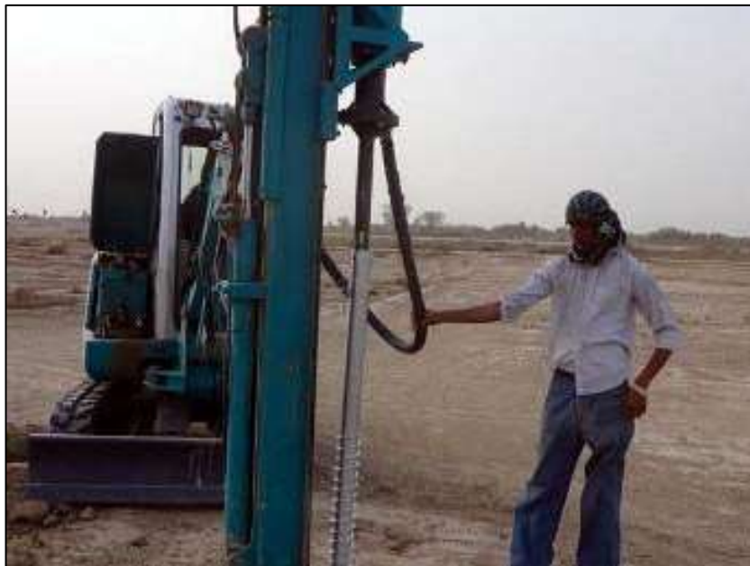
Figure 6: Ground Screw (Bulskop PV (Pty) Ltd, 2022)
