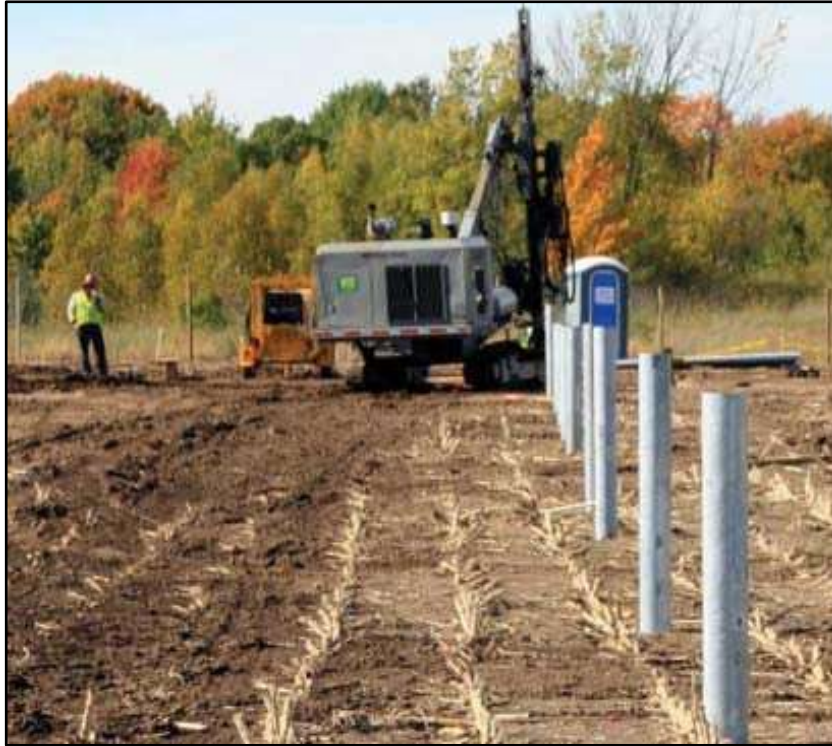
Figure 5: Driven/ Rammed Steel Pile (Bulskop PV (Pty) Ltd, 2022)
