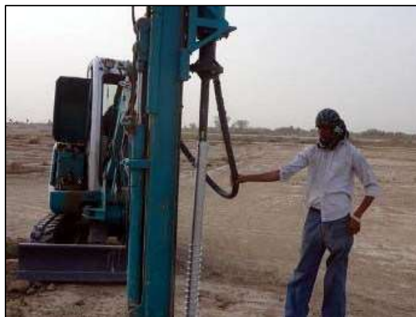
Figure 8: Ground Screw
