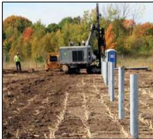
Figure 7: Driven/ Rammed Steel Pile
