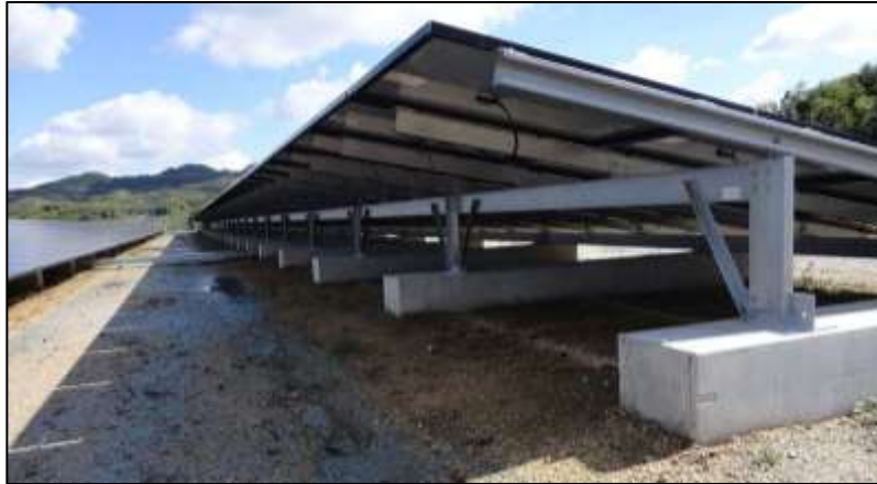
Figure 6: Cast Concrete Foundation
