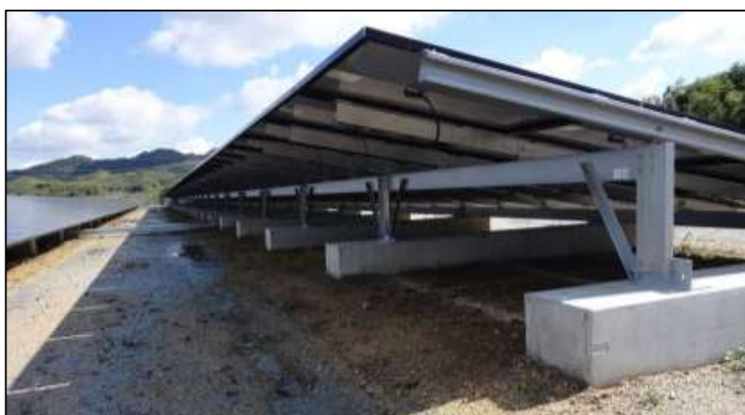
Figure 4: Cast Concrete Foundation (Gamka PV (Pty) Ltd, 2022).
