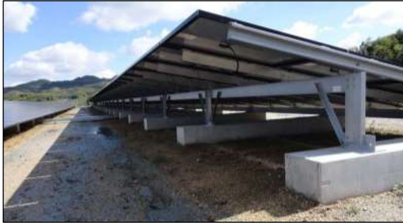
Figure 4: Cast Concrete Foundation
