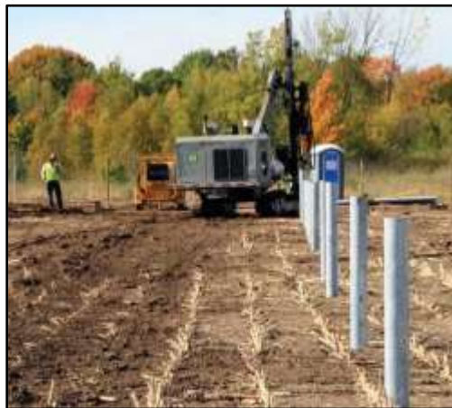
Figure 5: Driven/ Rammed Steel Pile
