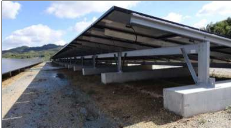
Figure 4: Cast Concrete Foundation
