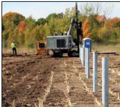
Figure 5: Driven/ Rammed Steel Pile
