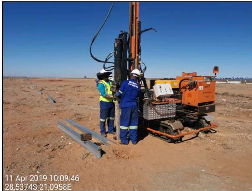
Figure 9: Ramming of steel piles into the pre-drilled / backfilled holes.
