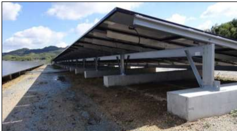
Figure 4: Cast Concrete Foundation (Salsola PV (Pty) Ltd, 2022).
