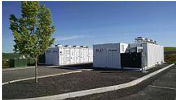
1 MW 4 MWh containerized vanadium flow battery owned by Avista Utilities and manufactured by UniEnergy Technologies
