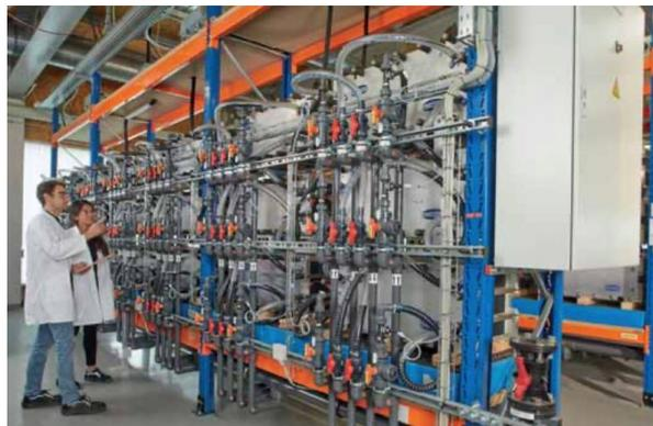
Stacks of a 2MW/20MWh vanadium redox flow battery at Fraunhofer ICT. Image:
