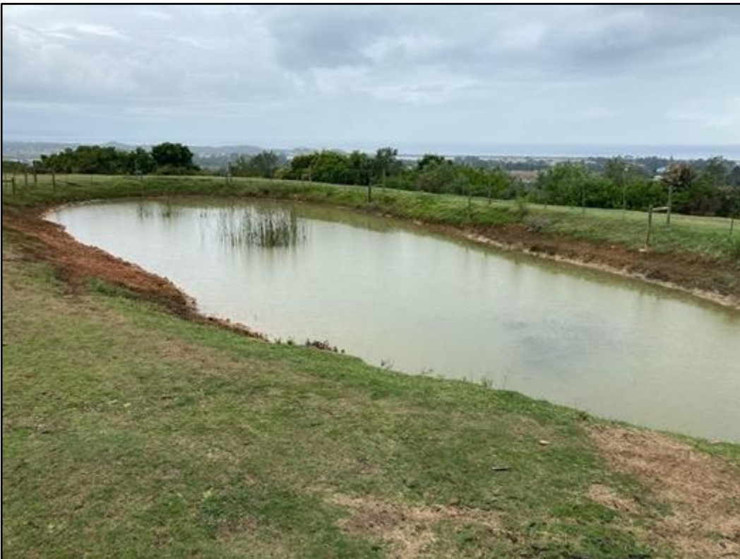
Figure 14: Small dam near top of slope on site.
