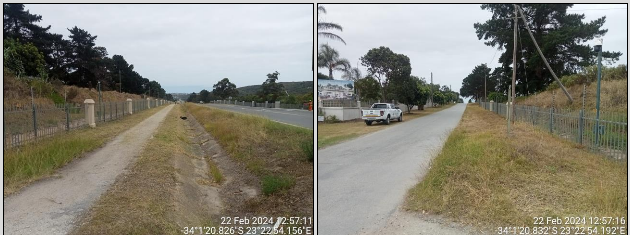
Figure 4: N2 road reserve (left) and Rietvlei Road road reserve (right). Required sewage infrastructure to be installed within the transformed areas of the road reserve.
