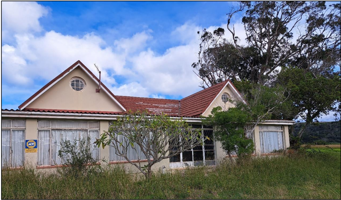
FIGURE 10: EXISTING RESIDENTIAL DWELLING
