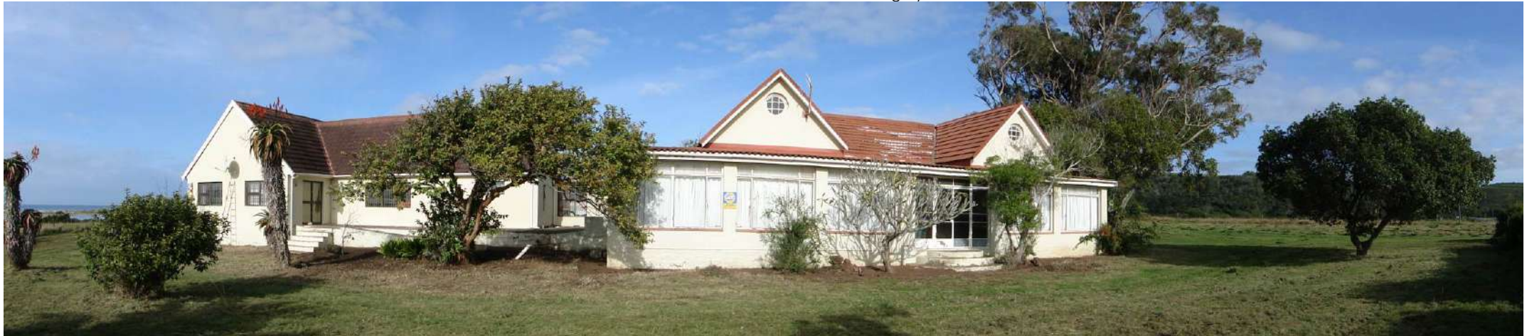
Photo 12: Northeast-facing elevation showing the historic homestead (right) and the modern home (left), which is physically connected to the historic homestead.
