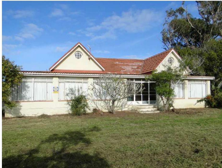
Photo 15: Historic core of historic homestead with enclosed stoep.
