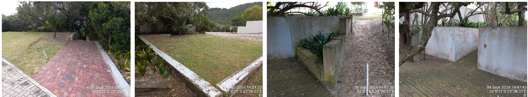
Figure 3: Photos of existing paved walkway & deck (on RE/106/304) & retained lawn & planter boxes on 118/304.
