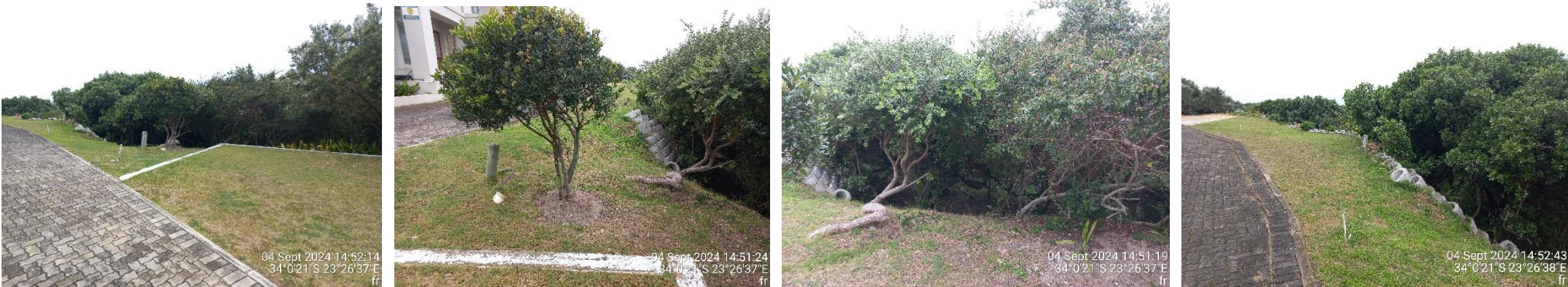
Figure 18: Views along northern boundary & existing retaining structures of 118/304. Note Milkwood below loffelstein, to be trimmed.
