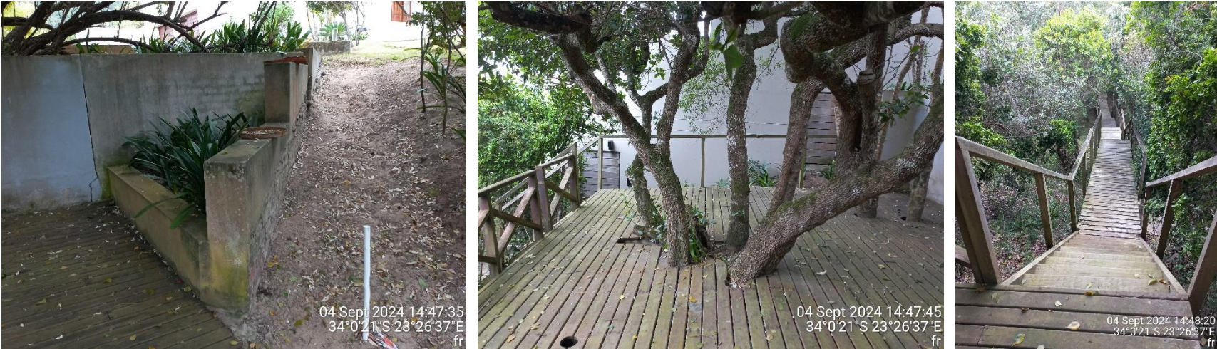
Figure 17: Retaining planter boxes, deck & boardwalk to beach on 106/304.
