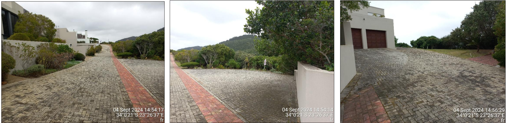
Figure 12: Paved Estate internal road, with paved parking area outside Erf 195 & wide driveway to existing double garage.
