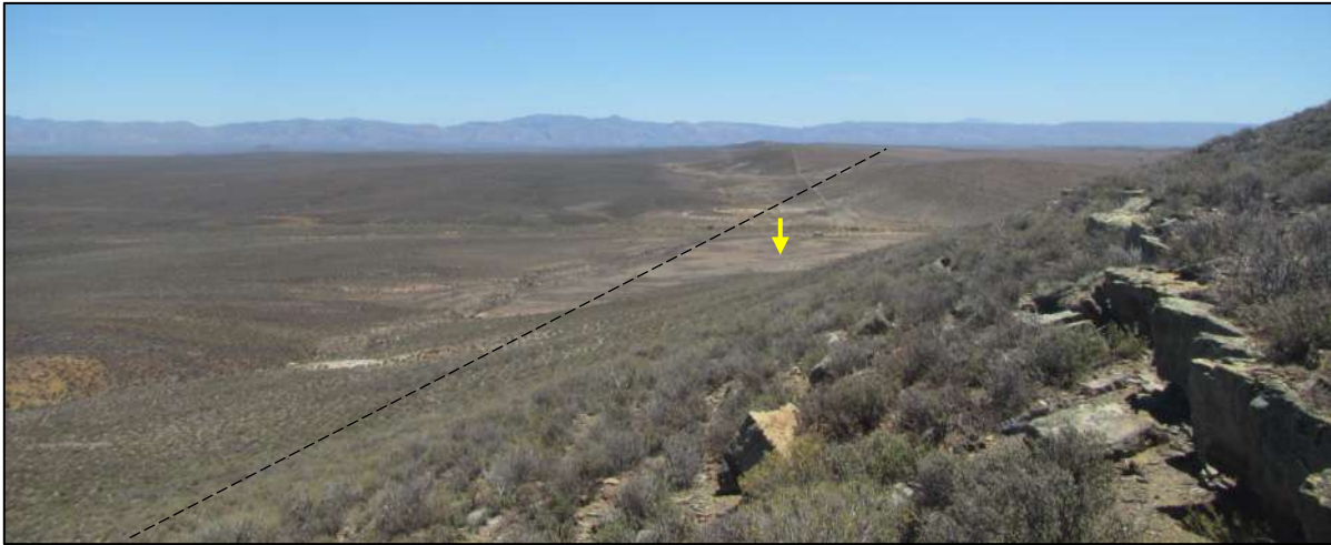
Figure 11: View towards the west from the eastern end of the west-east section of the power line corridor. The dashed line shows the approximate centre of the corridor until it passes over the ridge in the distance. The yellow arrow marks the location of Figure 12. Photographed 28 January 2020.
