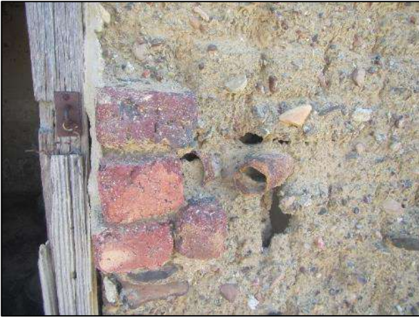
Figure 45: Detail of door frame and metal pipes supporting the internal hearth inside the cottage at waypoint 203.
