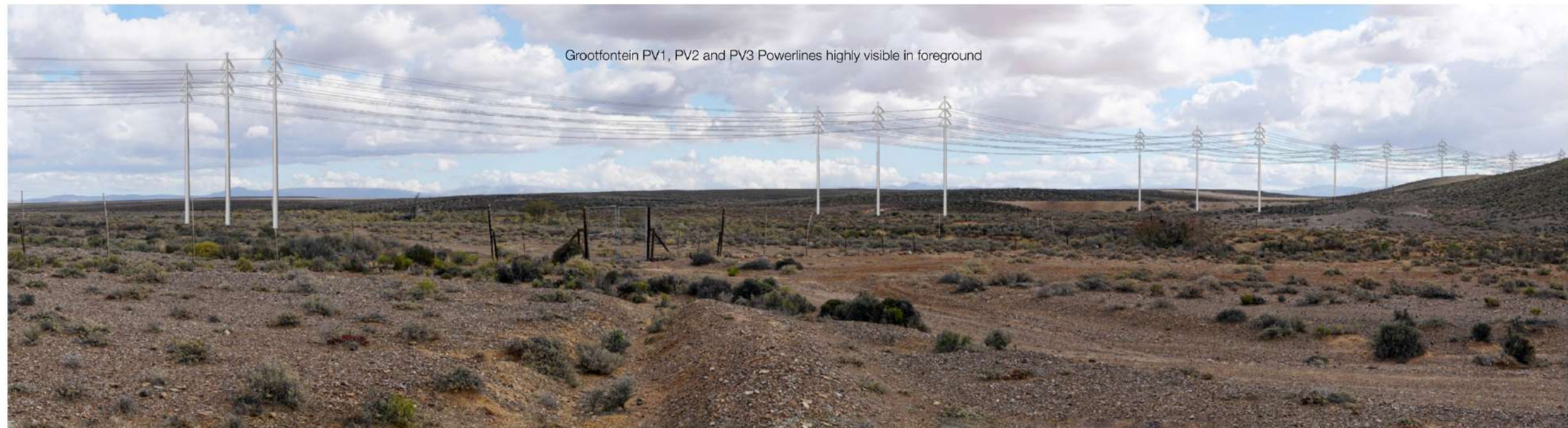
Viewpoint P2 : looking South-West from Wittewall Gate at Powerline Crossing
