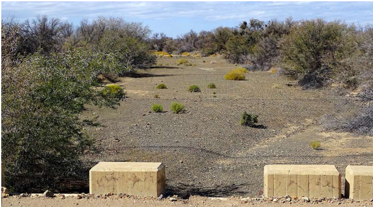
Figure 3: Dry riverbed of Groot River at the R356 road crossing
