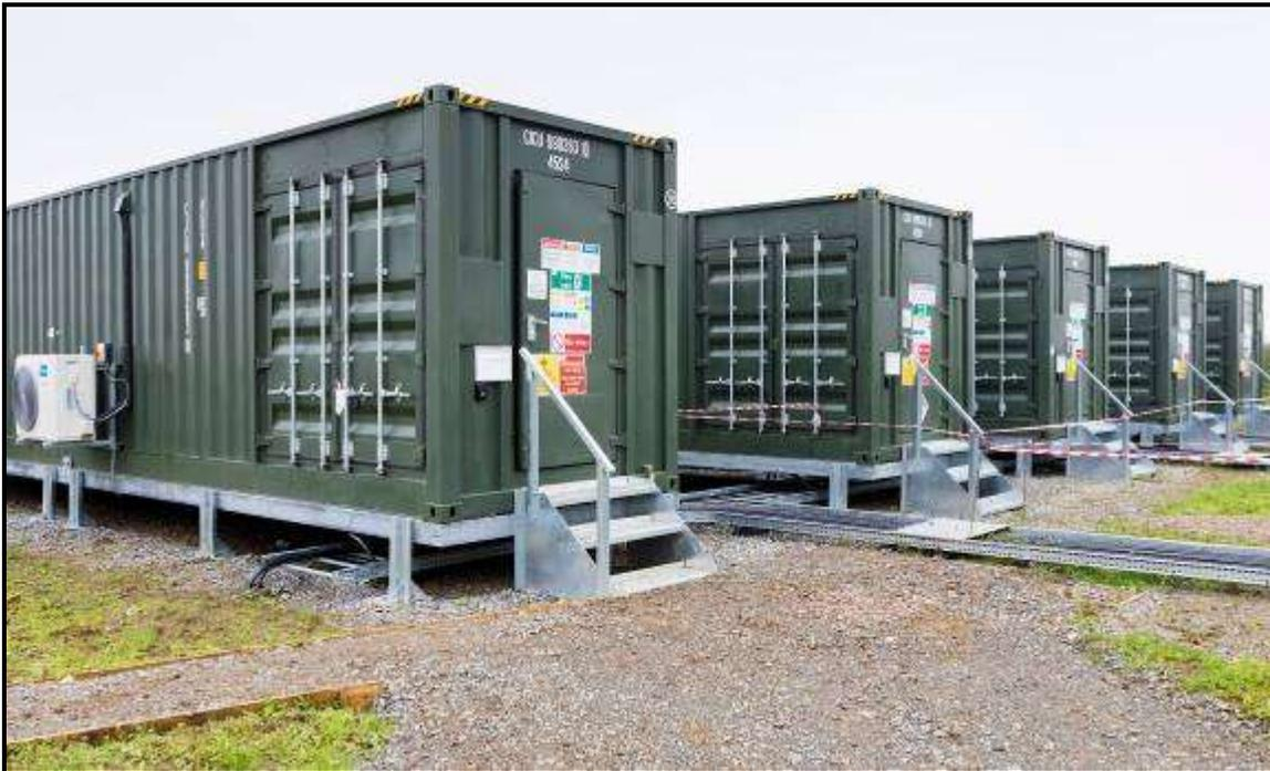
**Figure 1.3: Example of BESS located in storage containers**
