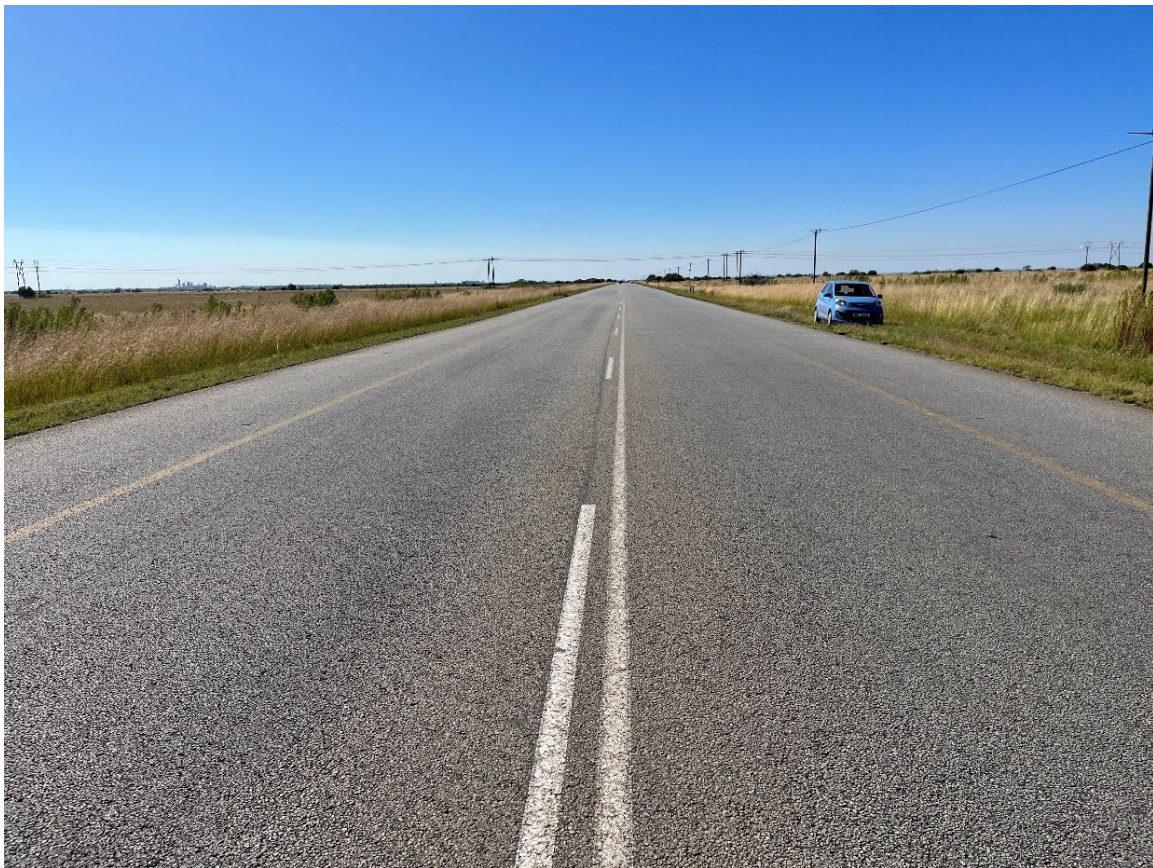
Figure 7.6 Existing Road P28-4 @ Km 7.15 – East Approaching (Access 1)
