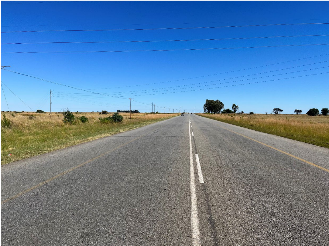
Figure 7.7 Existing Road P28-4 @ Km 7.15 – West Approaching (Access 1)
