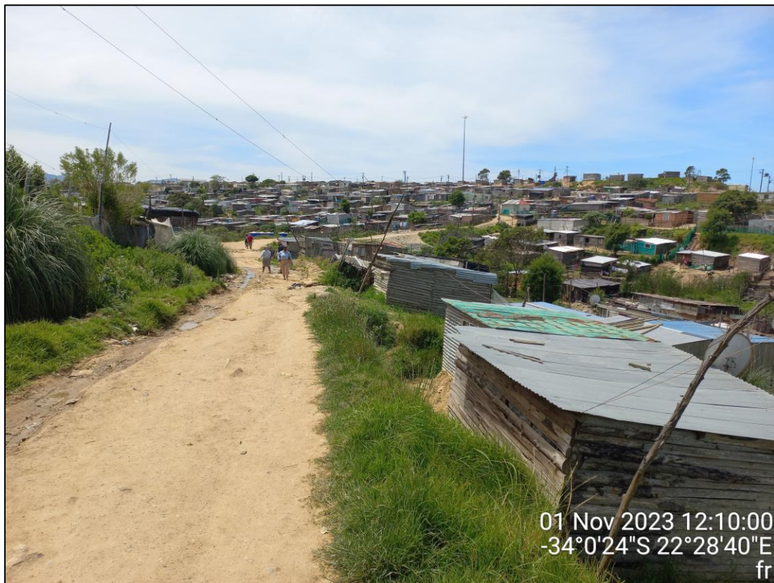
Figure 4: Informal houses erected over the approved sewer pipeline route since the issue of the Environmental Authorisation in 2014.
