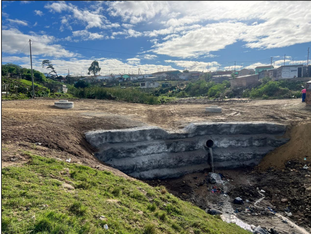
Figure 19: Newly constructed gabion wall. Reno mattresses proposed at the foot of the gabion wall to prevent erosion from plunging water in the stream bed. Reno mattress proposed above the gabion wall to prevent erosion caused by blocked stormwater pipelines causing water to flow over the face of the gabion wall.
