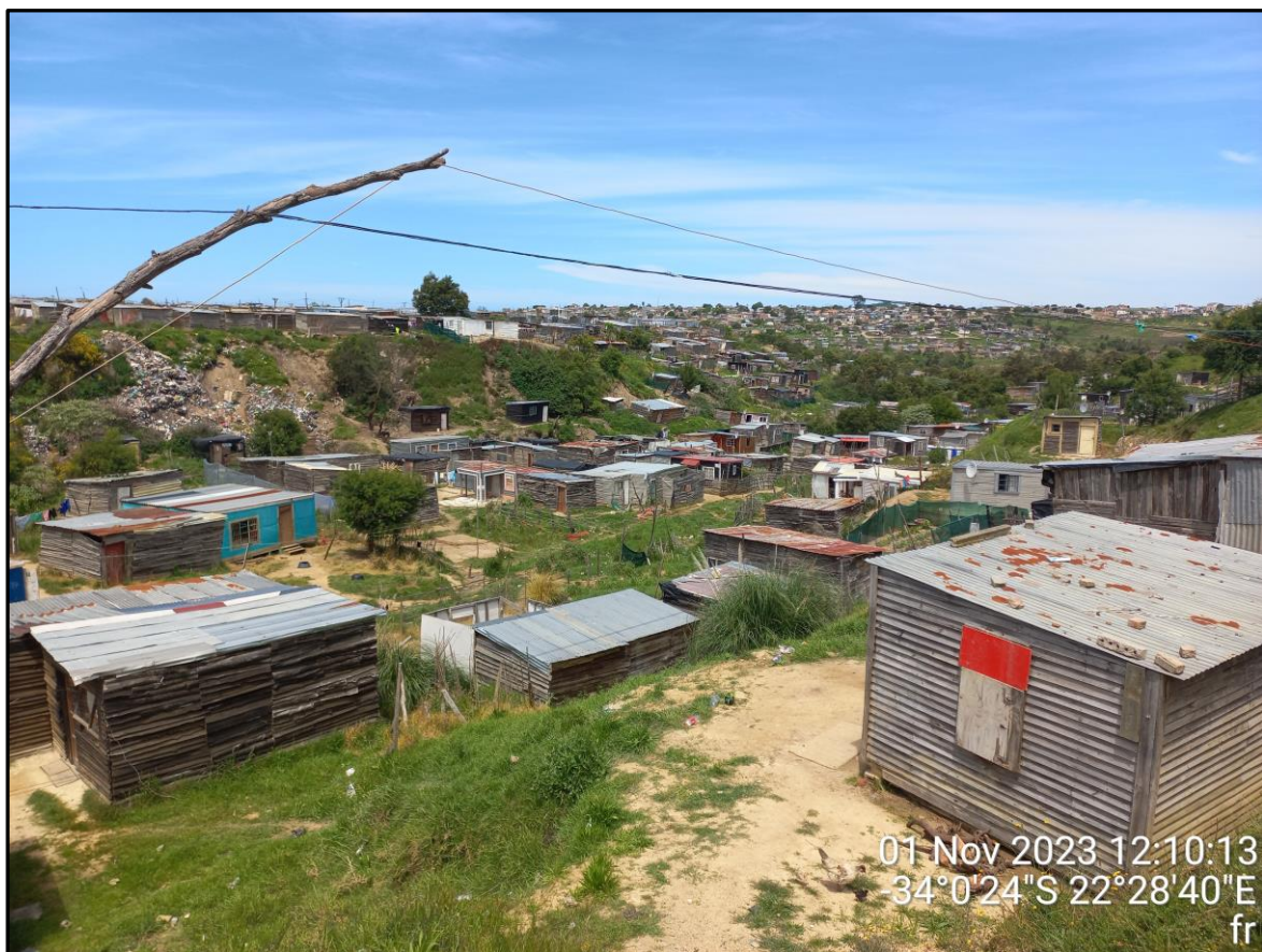
Figure 7: Steep slopes and informal housing units located in close proximity to the proposed pipeline route.
