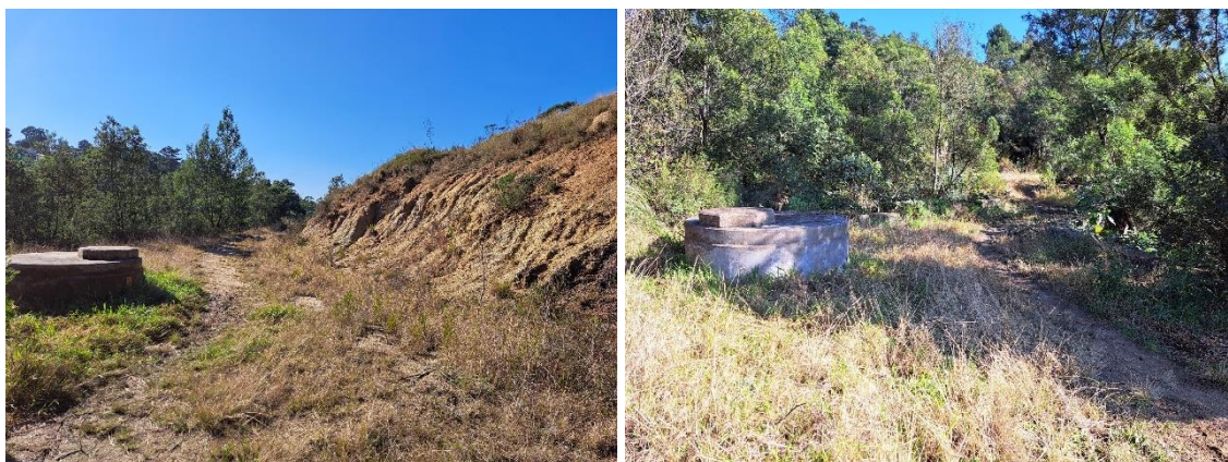
Figure 3. Example of the bulk sewer line installed on the opposite side of the Skaapkop River in Pacaltsdorp where the sewerline has become a single lane dirt track following benching.
