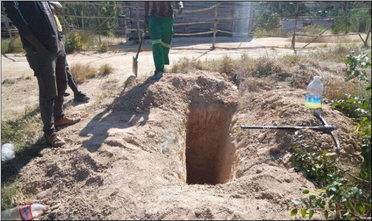
Figure 13: Test pits conducted on site
