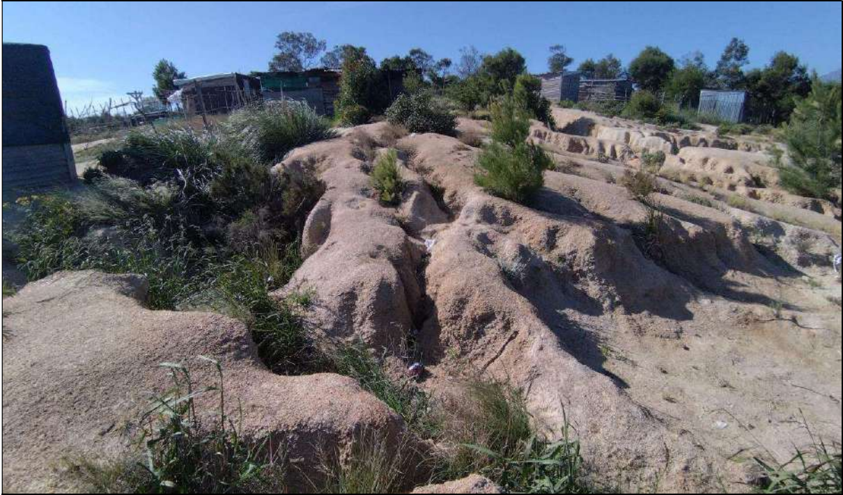
Figure 10: Erosion dongas commonly seen on the site
