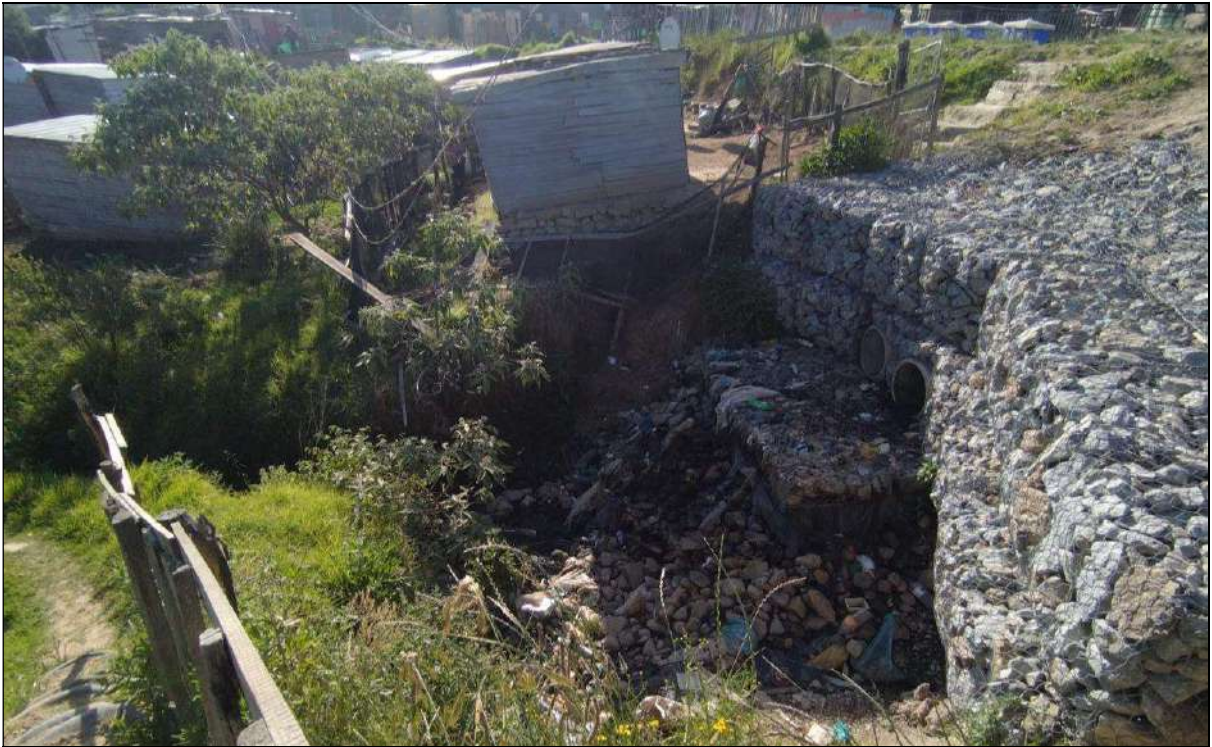
Figure 7: Existing stormwater pipe culvert near TP4
