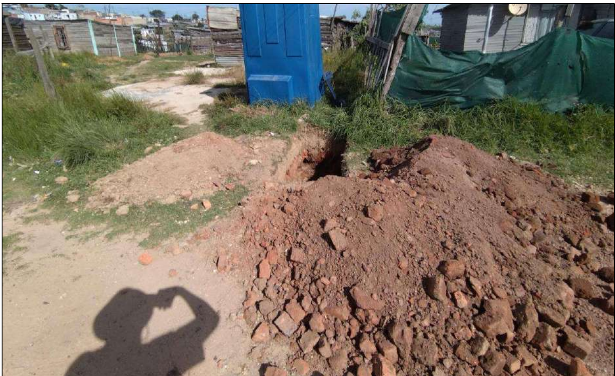
Figure 15: Brick rubble fill encountered at TP1
