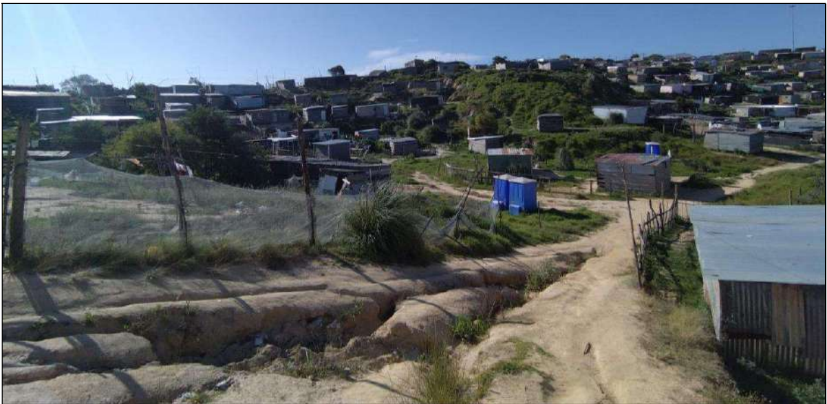
Figure 5: Footpaths on site
