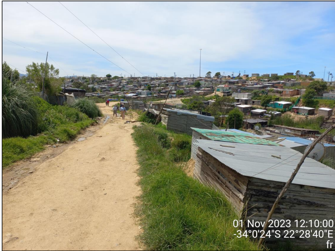
Figure 4: Informal houses erected over the approved sewer pipeline route since the issue of the Environmental Authorisation in 2014.
