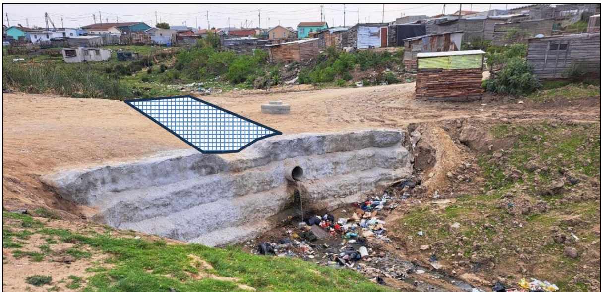
Figure 20: Schematic drawing of the proposed Reno mattress above the gabion wall to prevent erosion caused by blocked stormwater pipelines causing water to flow over the face of the gabion wall (Confluent Environmental, 2024).
