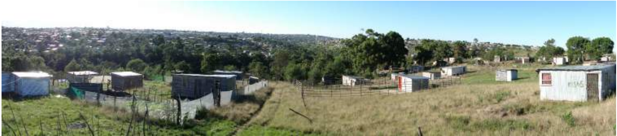
Photo 3: South-facing view, western half of study area, Schaapkop River in background. Proposed bulk sewer line to largely follow the outer edge of existing settlement.
