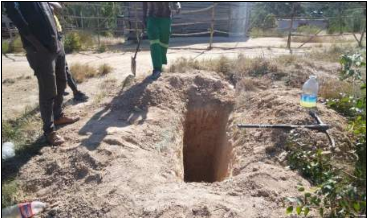
Figure 13: Test pits conducted on site
