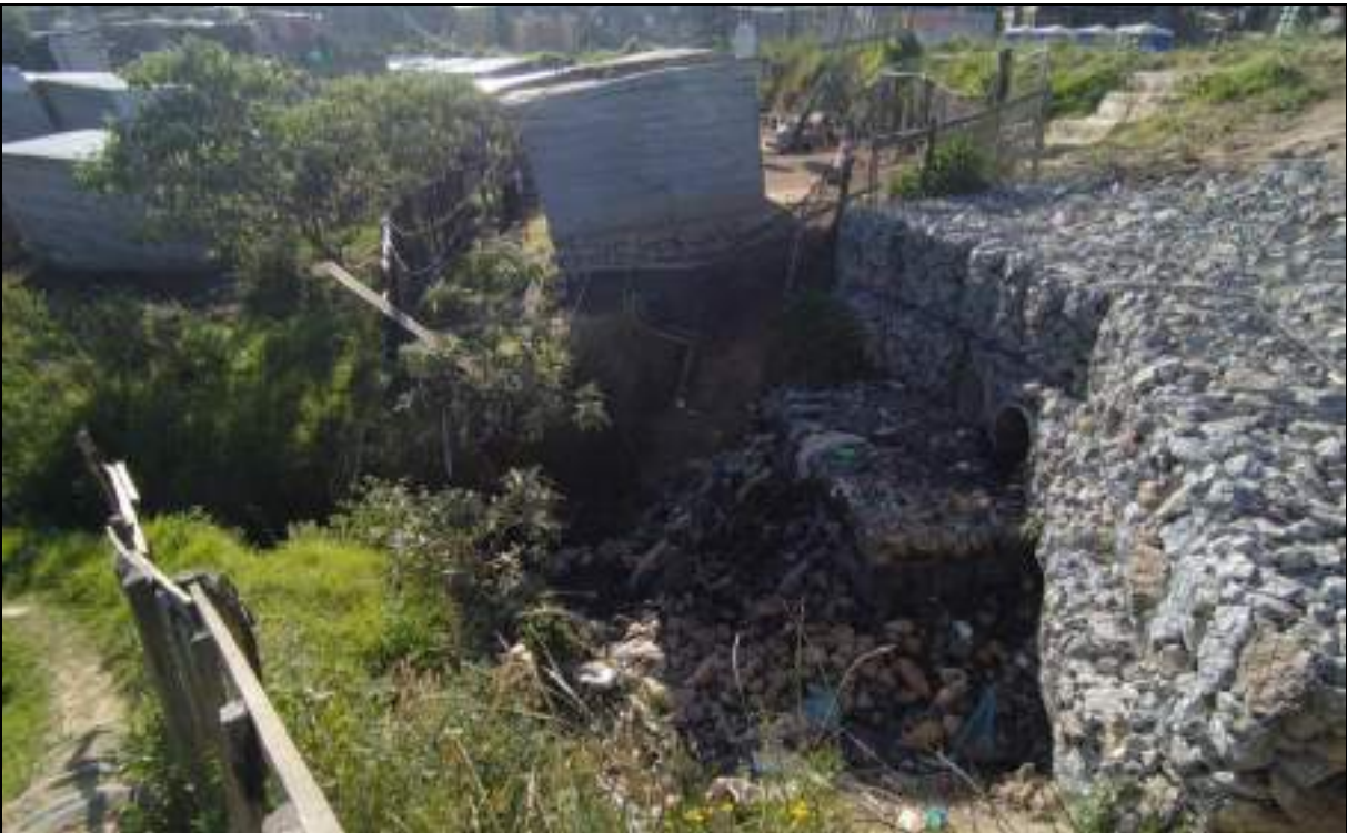
Figure 7: Existing stormwater pipe culvert near TP4
