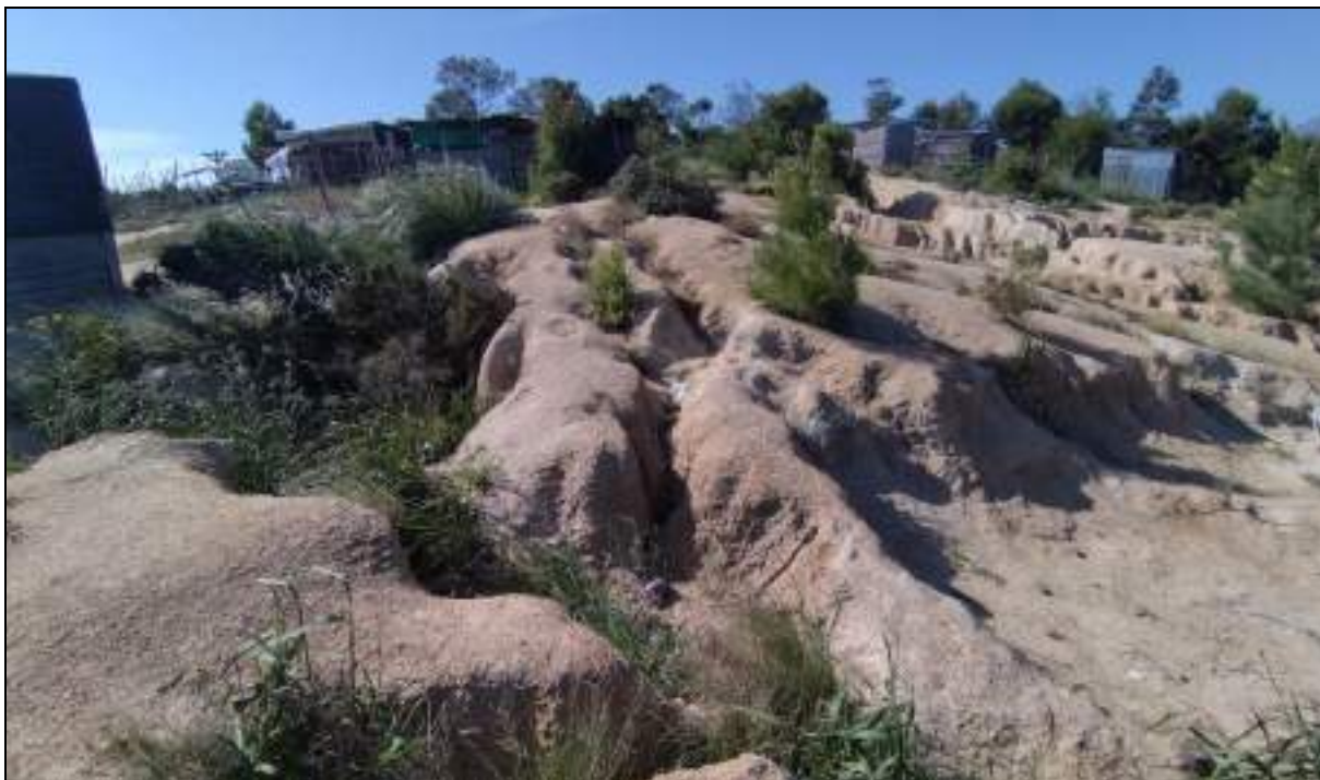
Figure 10: Erosion dongas commonly seen on the site
