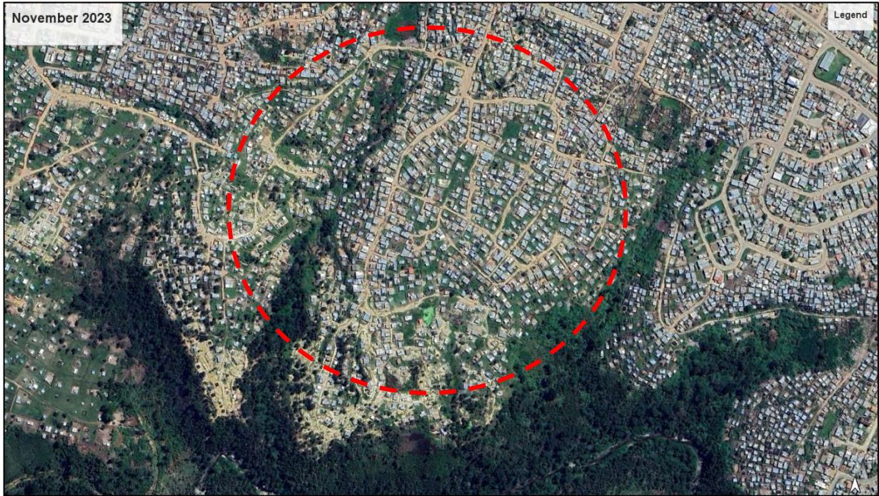
Figure 3: Aerial imagery of the old 'All Brick' brickworks site in 2023 (Google Earth, 2024).
