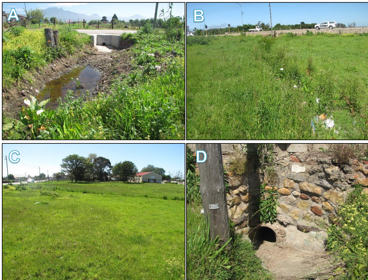
Figure 5: Photographs from the site including the stormwater headwall discharging into the channel from Church Street (A); view of the channel in the direction of Beach Road (B); view of the channel from Beach Road (C); and the culvert that conveys stormwater flows from the channel beneath Beach Road (D).
