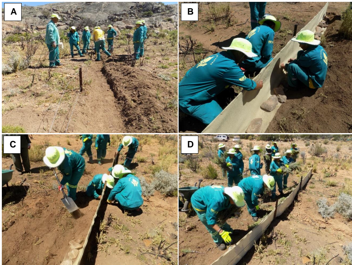
Figure 7. Installation of the soil erosion control fence. A: Installing the standards and wires and preparing the trench. B: Fitting the geotextile, tying it on with wire. C: Filling in the trench over the geotextile. D: Applying a mulch against the completed fence (Photos courtesy Ken Coetzee).
