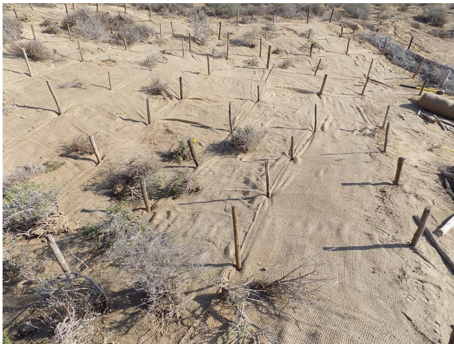
Figure 9. Example of how Soilsaver is fitted to the soil surface (Photo courtesy Ken Coetzee). Note holes to accommodate indigenous vegetation.
