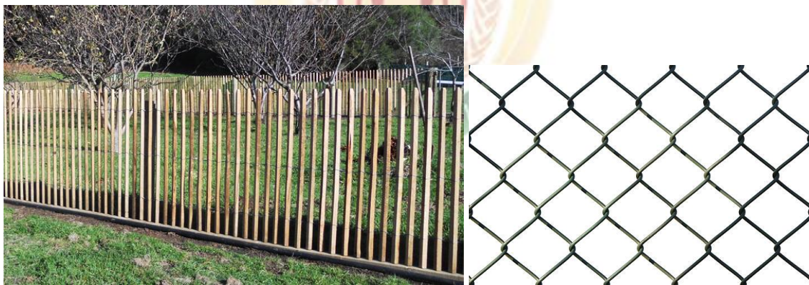
Figure 4:.. Suggested fencing showing wood lattice for aesthetic appeal, approximate spacing so the wetland is visible, and diamond mesh which must be on the inside of wooden lattice.
