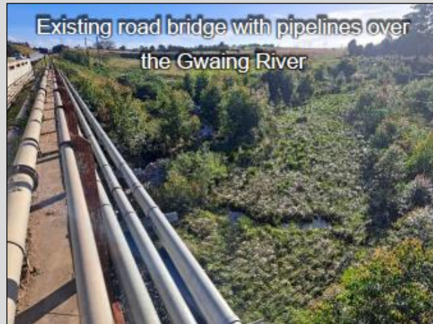
Figure 6: Gwaing River bridge with existing pipelines.
