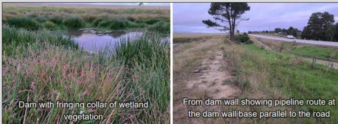
Figure 13: Crossing D – Dam embankment with road parallel (source: Confluent).
