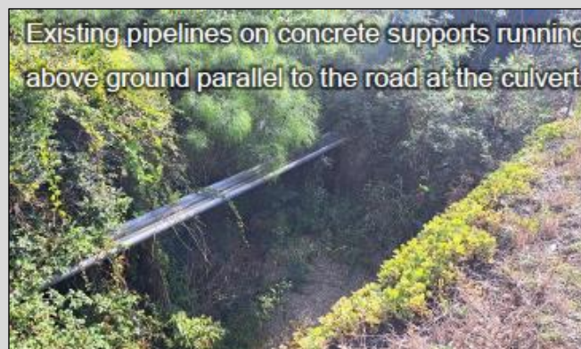
Figure 7: Norga River culvert crossing.
