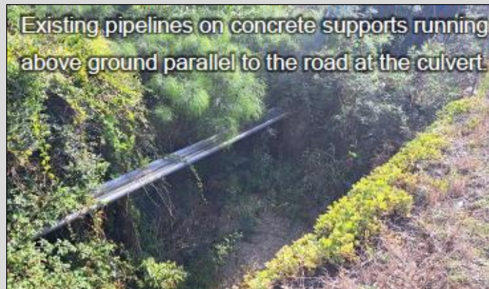
Figure 4: Norga River culvert crossing.
