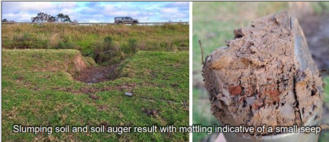
Figure 12: Crossing C – Seep Wetland.
