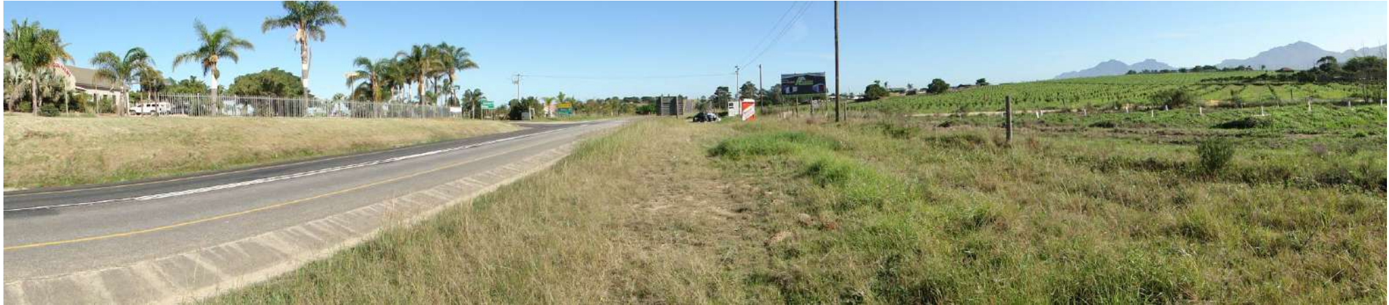
Photo 5: West-facing view – proposed pipeline alignment to be installed within road reserve to right of R102 as seen in this image.
