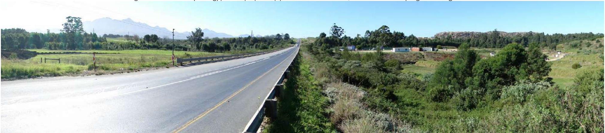
Photo 2: East facing view (towards George/ York Street) from western side of Gwayang River bridge.
