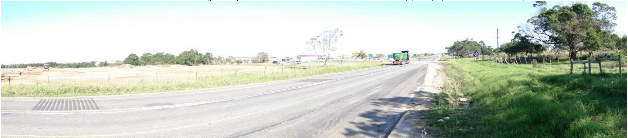
Photo 12: West-facing view towards R102 and Blanco Road intersection with George Airport in the background. Proposed pipeline proposed to cross R102 (right to left on this image) at this point.
