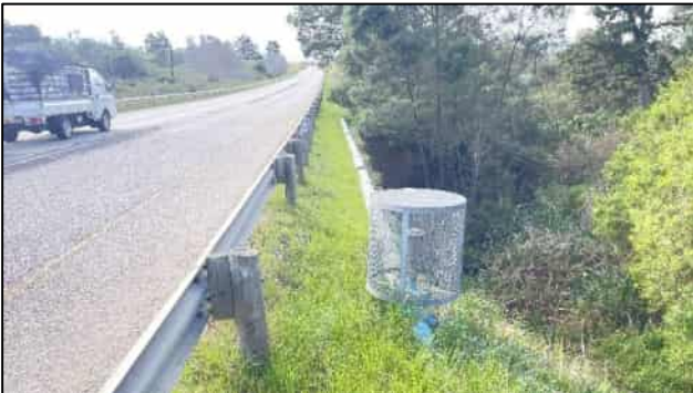
Figure 4-2: Existing Culvert Crossing
