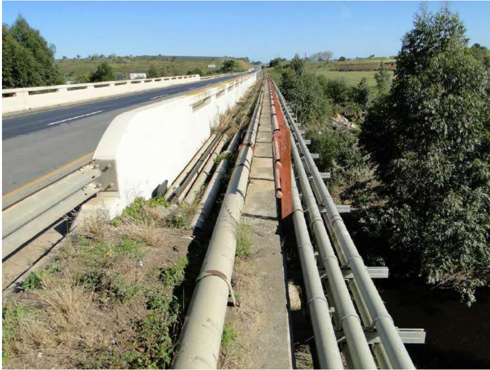
Photo 3,4: New water pipeline to be affixed to Gwayang River bridge noted in two images above.
