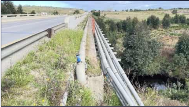
Figure 4-1: Existing Bridge Crossing
