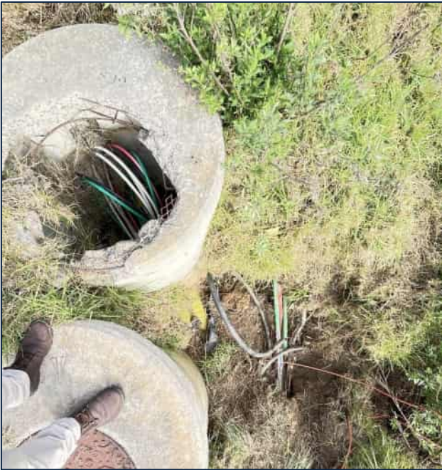
Figure 3-4: Fibre Manhole
