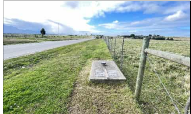
Figure 3-3: Existing Sewer Pipeline
