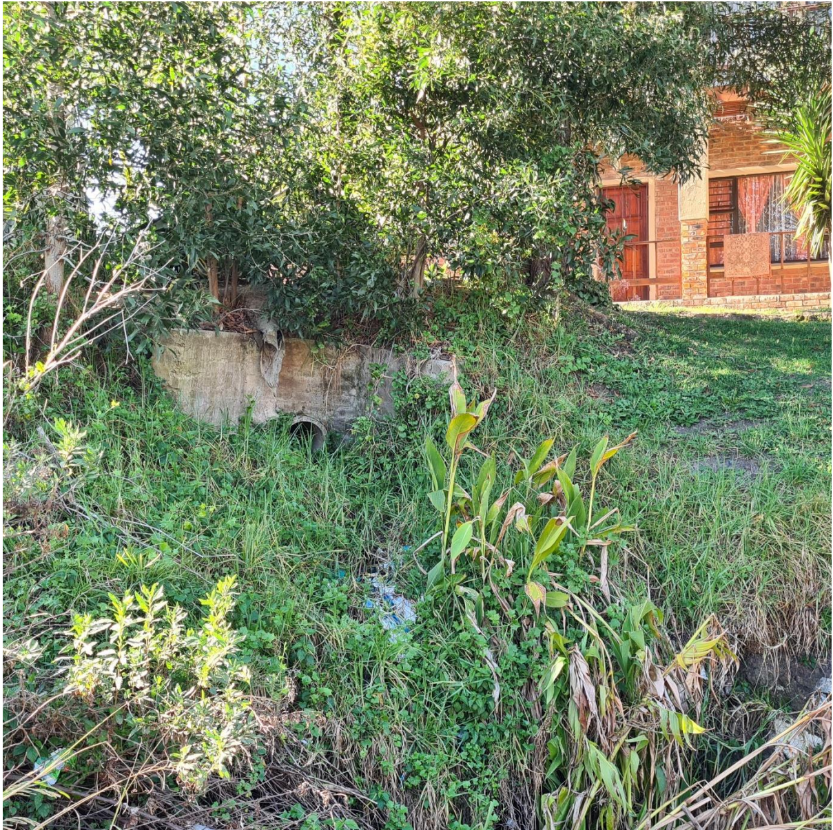
Figure 4: Stormwater outlet along Erf 21150.
