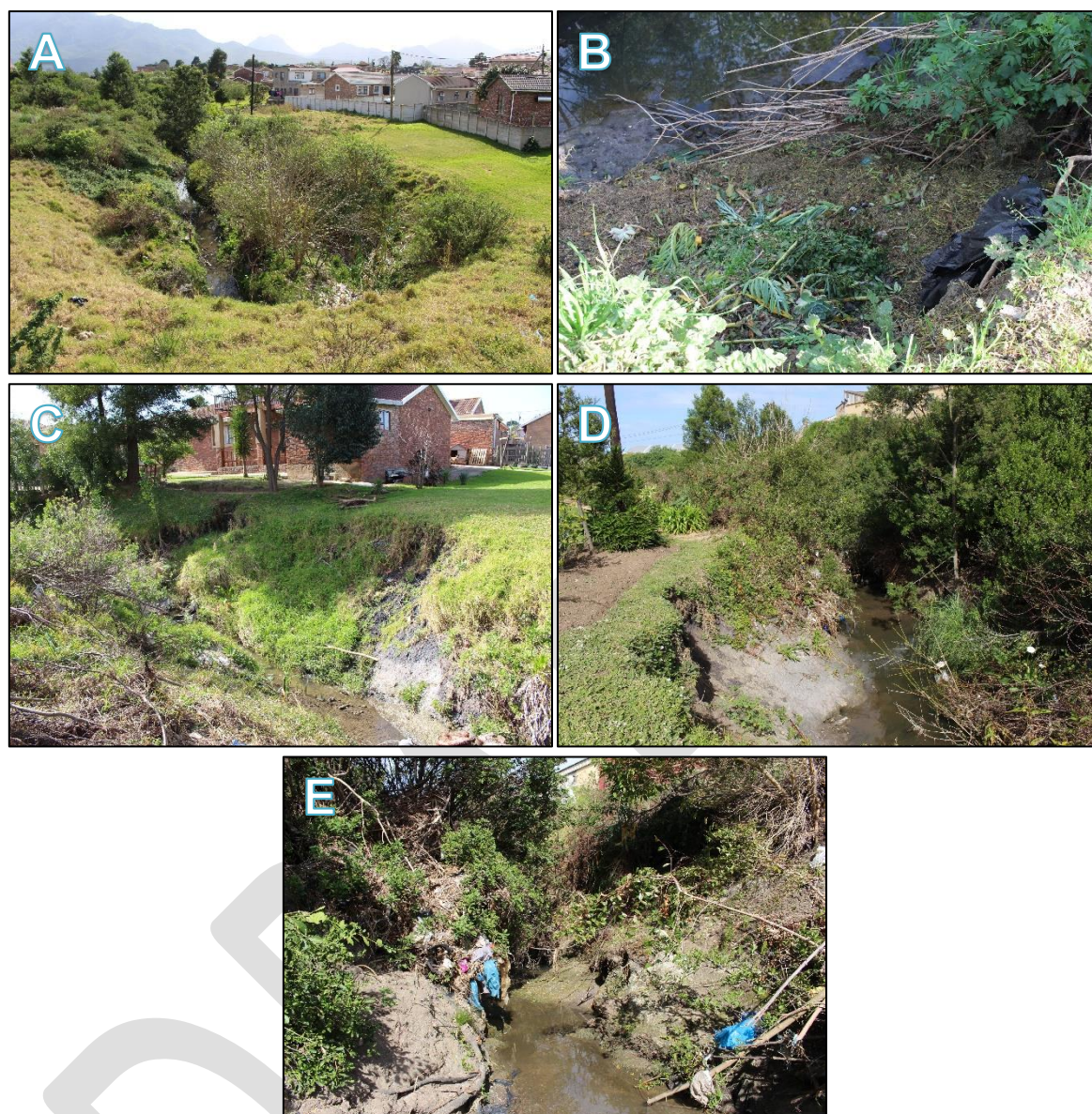
Figure 4: View of the wetland looking north from Grens Road (A); dumping of litter and garden waste into the wetland (B); eroded banks adjacent to Erf 21151 (C); erosion of banks in-stream habitat and eroded banks of the wetland (top) and eroded channel adjacent to erfven 21150 and 21151 (bottom).
