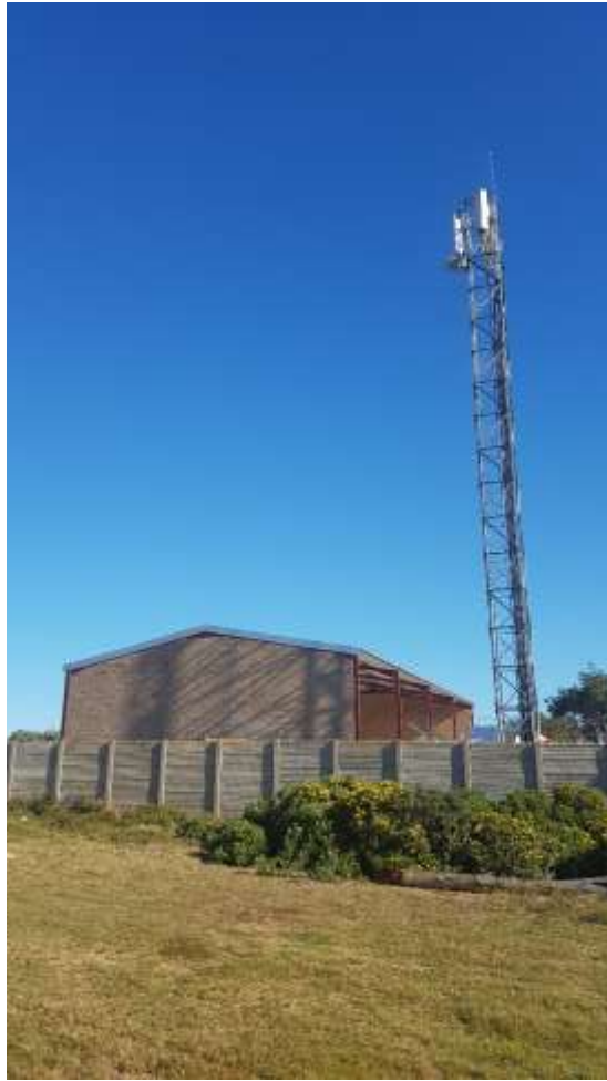
Figure 7: Existing structure along the south-eastern boundary of the property.
