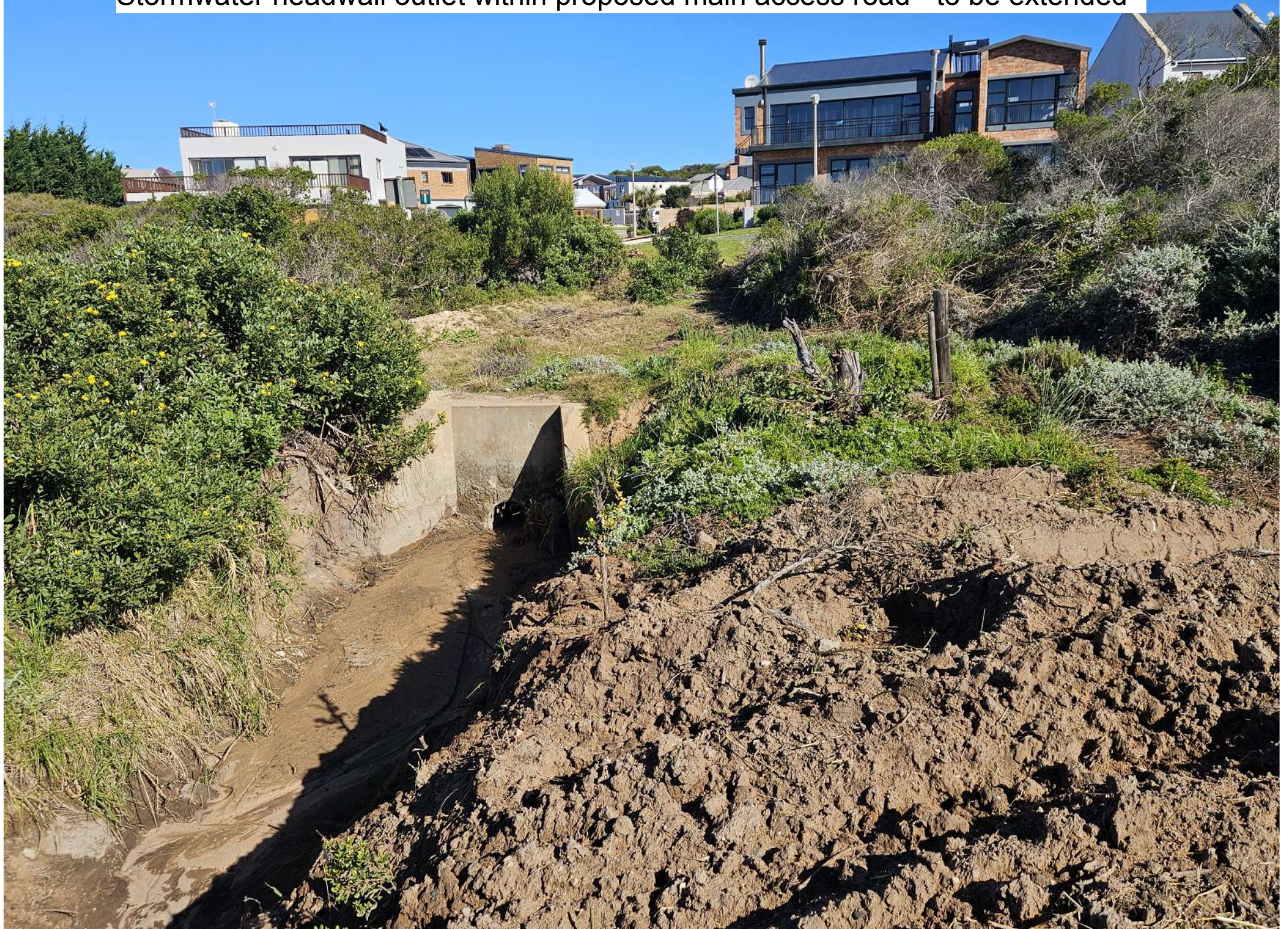
Stormwater headwall outlet within proposed main access road - to be extended
