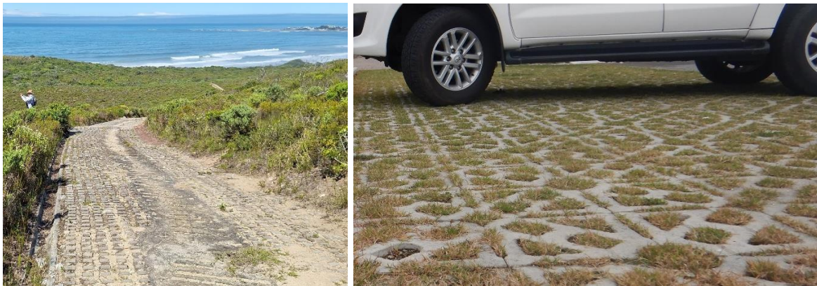
Figure 17: An image of roads associated with minimal edge effects.
