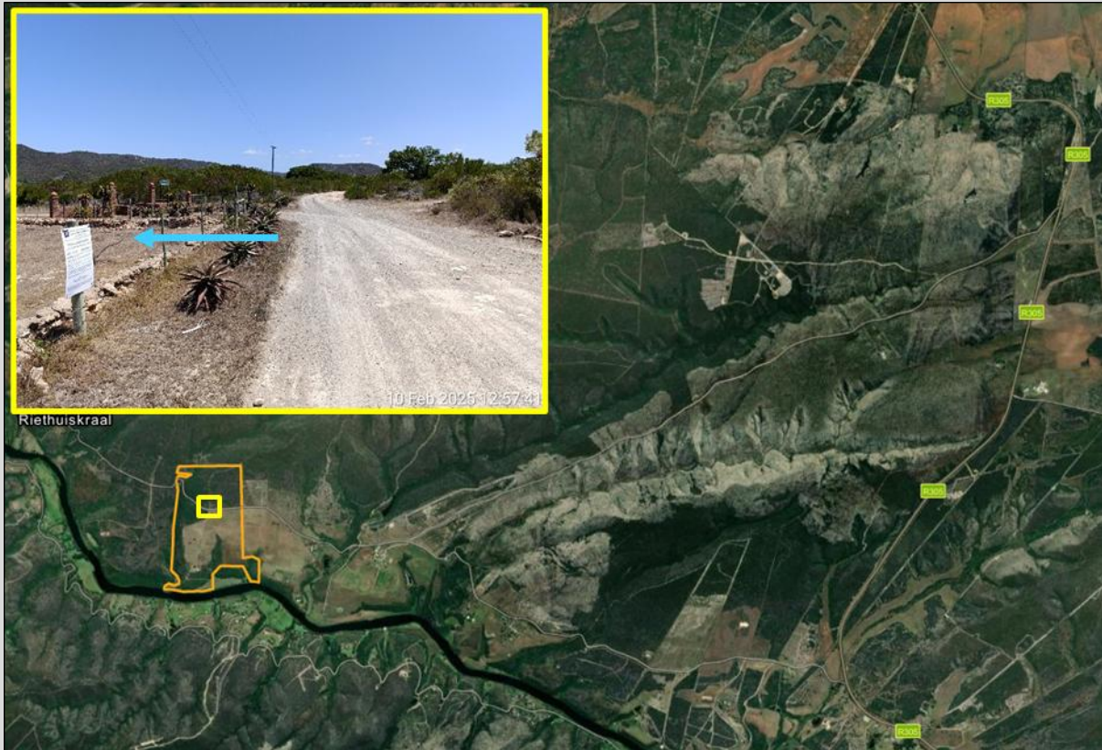
Figure 2: Existing access to Farm via a gravel road that connects directly to the R305. The yellow box within the farm property indicates the approximate locality of the photo above.
