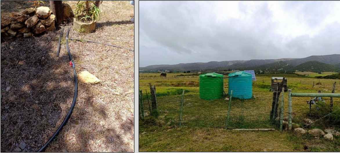
Figure 32: Existing surface-laid water pipeline at the neighbouring farm property (132/480) which receives water from an existing borehole on 257/480.
