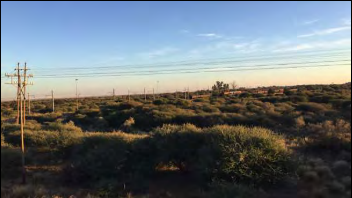
Figure 23: View north from Photo 5 of the existing power line and railway line infrastructure along which the proposed power line would be routed.
