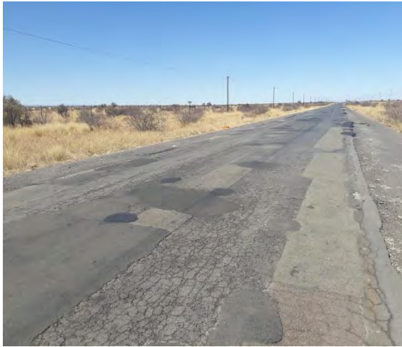
Photograph 3.3: Patching along the route
