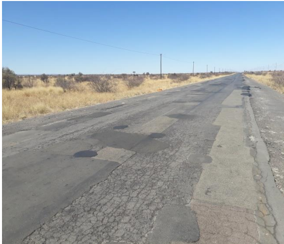
Photograph 3.3: Patching along the route
