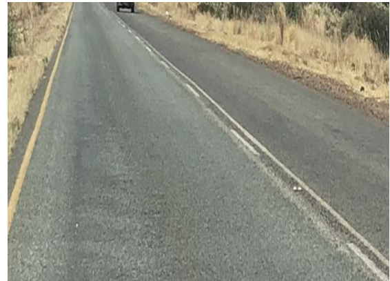
Photograph 3.2: Road markings on R31
