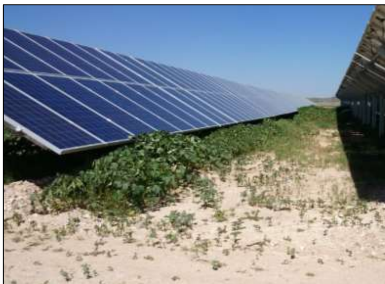
Figure 3: dense infestation of Stinkblaar ( Datura ferox ) growing at a South African solar PV plant shortly after construction. A large proportion of this invasion could have been avoided if the vegetation beneath the panels had not been cleared as this vegetation would have utilised the water running off the front of the panels and limited the invasion of the Datura .
