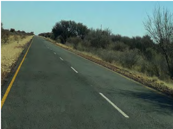
Photograph 3.1: Road condition R31
