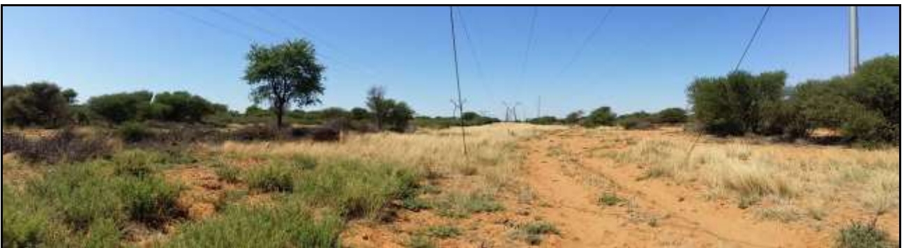
Figure 8: View in a southerly direction of the OHL crossing the eastern edge of Portion 11 of York A 279, belonging to Kudumane Manganese Resources (KMR).
