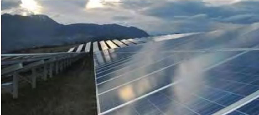
The design of the fittings for fixing the modules to the rack structures will enable thermal expansion of the metal without transferring mechanical loads that could affect the integrity of the modules. The structure will probably have anti-theft bolts.
