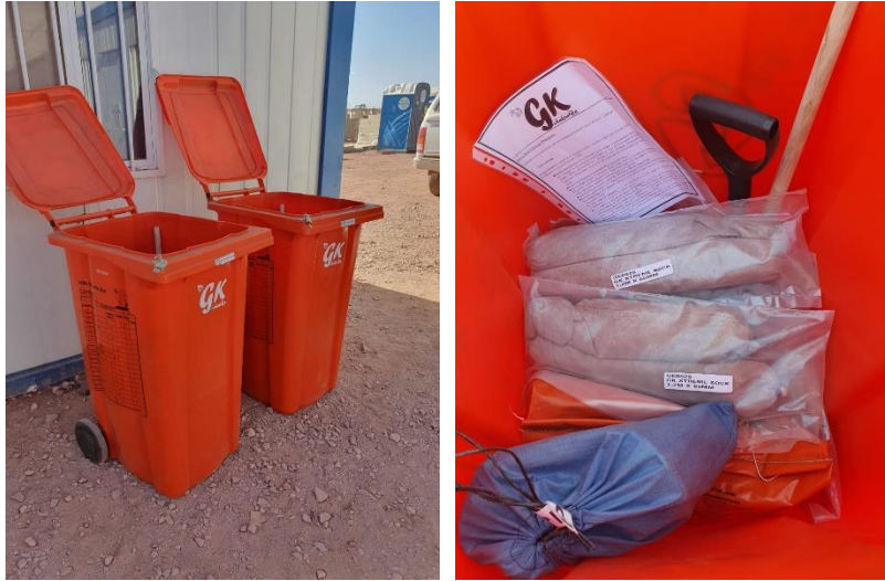
Figure 8: Example of a hydrocarbon Spill Kit to be in place within the site camp.
