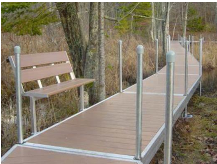
Figure 42: Example of modular lightweight boardwalk design allowing sections to be removed.
