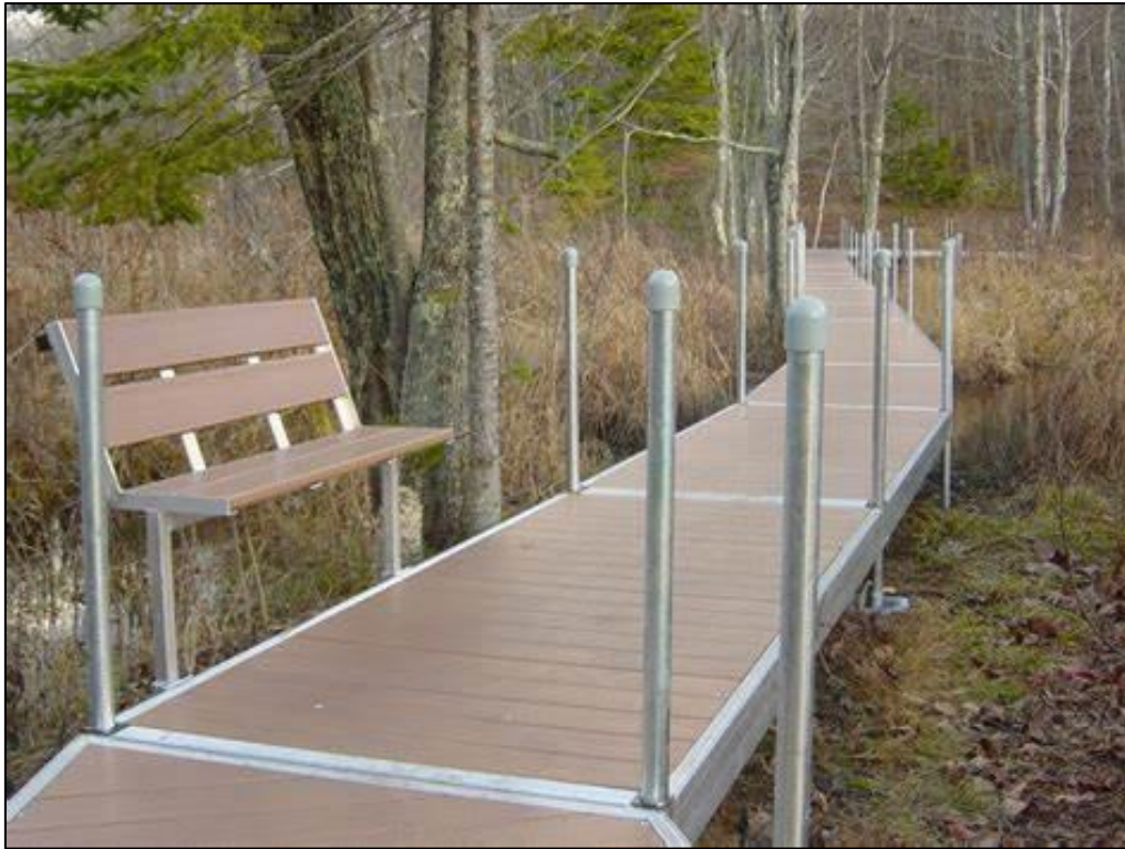
Figure 12: An image of a “modular aluminium boardwalk”, as an example of a lightweight board walk design where sections of the flat boardwalk can be easily removed from the site. This is an American company ( greatnortherndocks.com ), but a similar concept can be applied for the proposed tented camp at Diepwalle.
