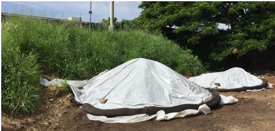
Figure 11: An example of a protected stockpile (image from stormwaterhawaii.com).
