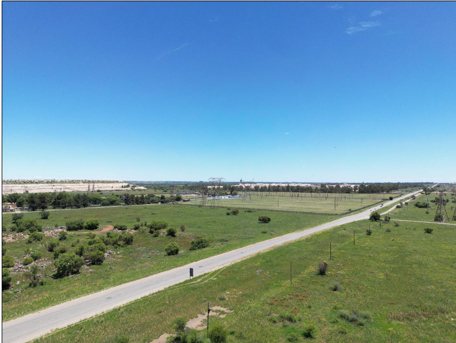
Figure 3.23: Aerial photo at Hermes Substation taken towards the south-west: AGL 30m
