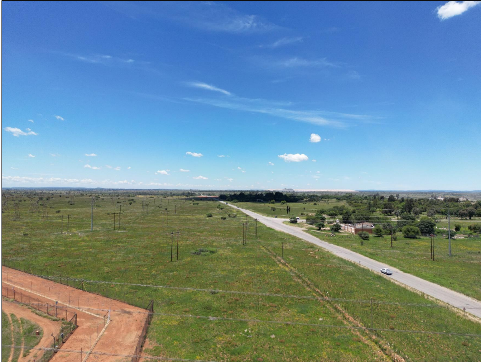
Figure 3.20: Aerial photo at Hermes Substation taken towards the east: AGL 30m
