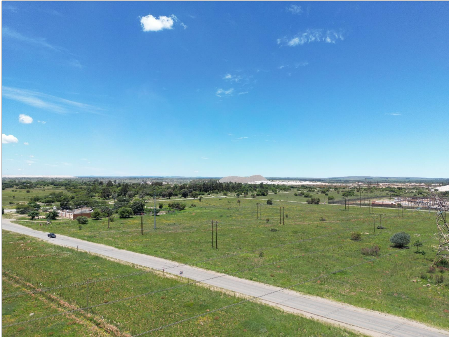
Figure 3.21: Aerial photo at Hermes Substation taken towards the south-east: AGL 30m
