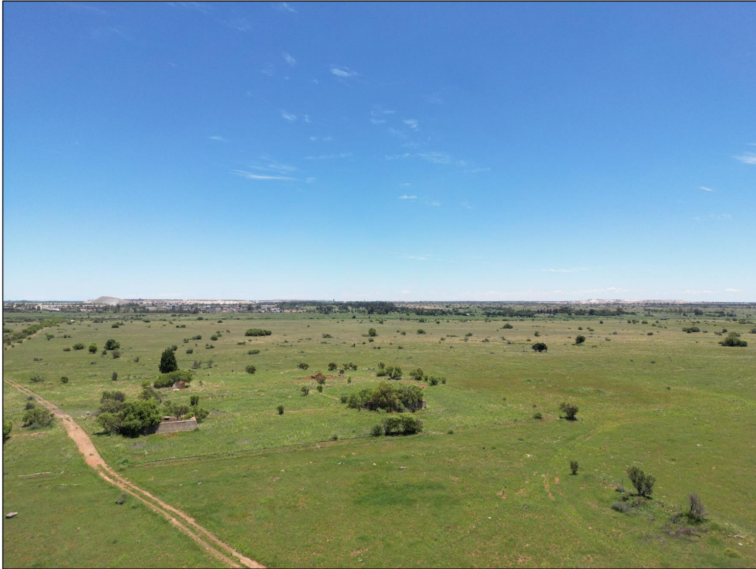
Figure 3.16: Aerial photo at Buffels East Substation taken towards the west: AGL 30m
