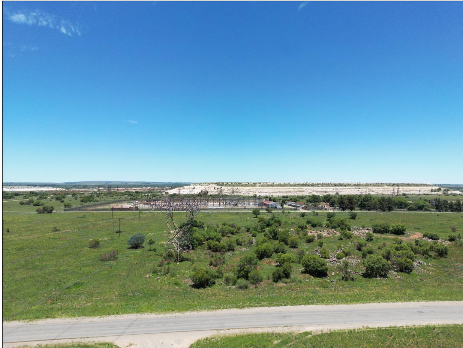
Figure 3.22: Aerial photo at Hermes Substation taken towards the south: AGL 30m
