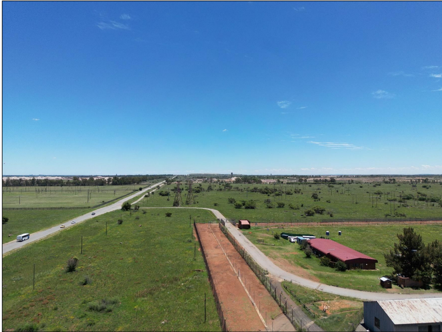
Figure 3.24: Aerial photo at Hermes Substation taken towards the west: AGL 30m
