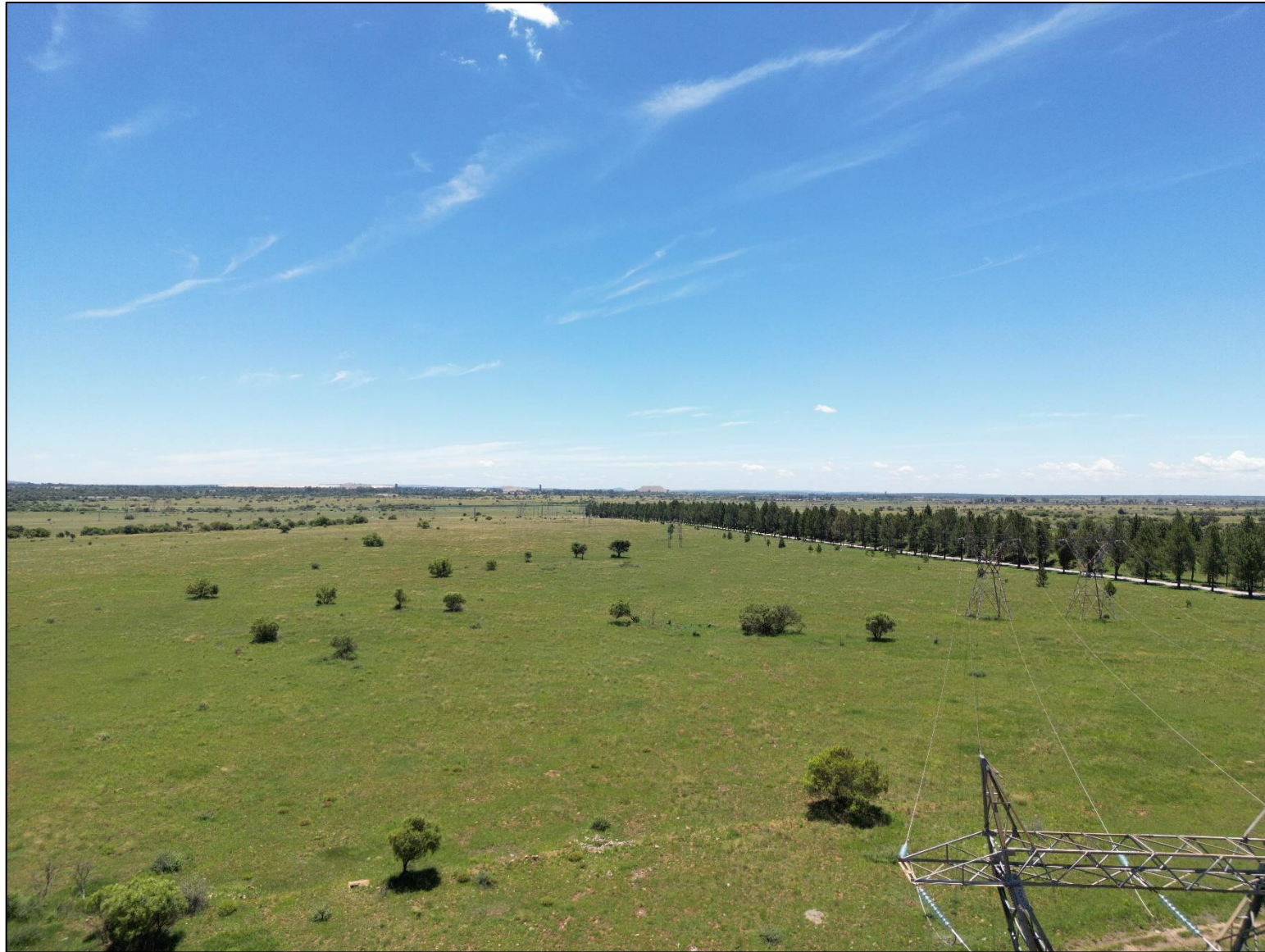
Figure 3.10: Aerial photo at Buffels East Substation taken towards the north: AGL 30m
