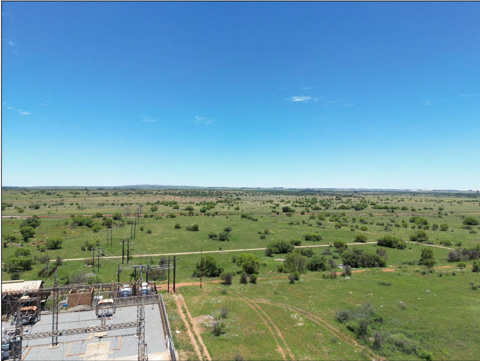
Figure 3.14: Aerial photo at Buffels East Substation taken towards the south: AGL 30m
