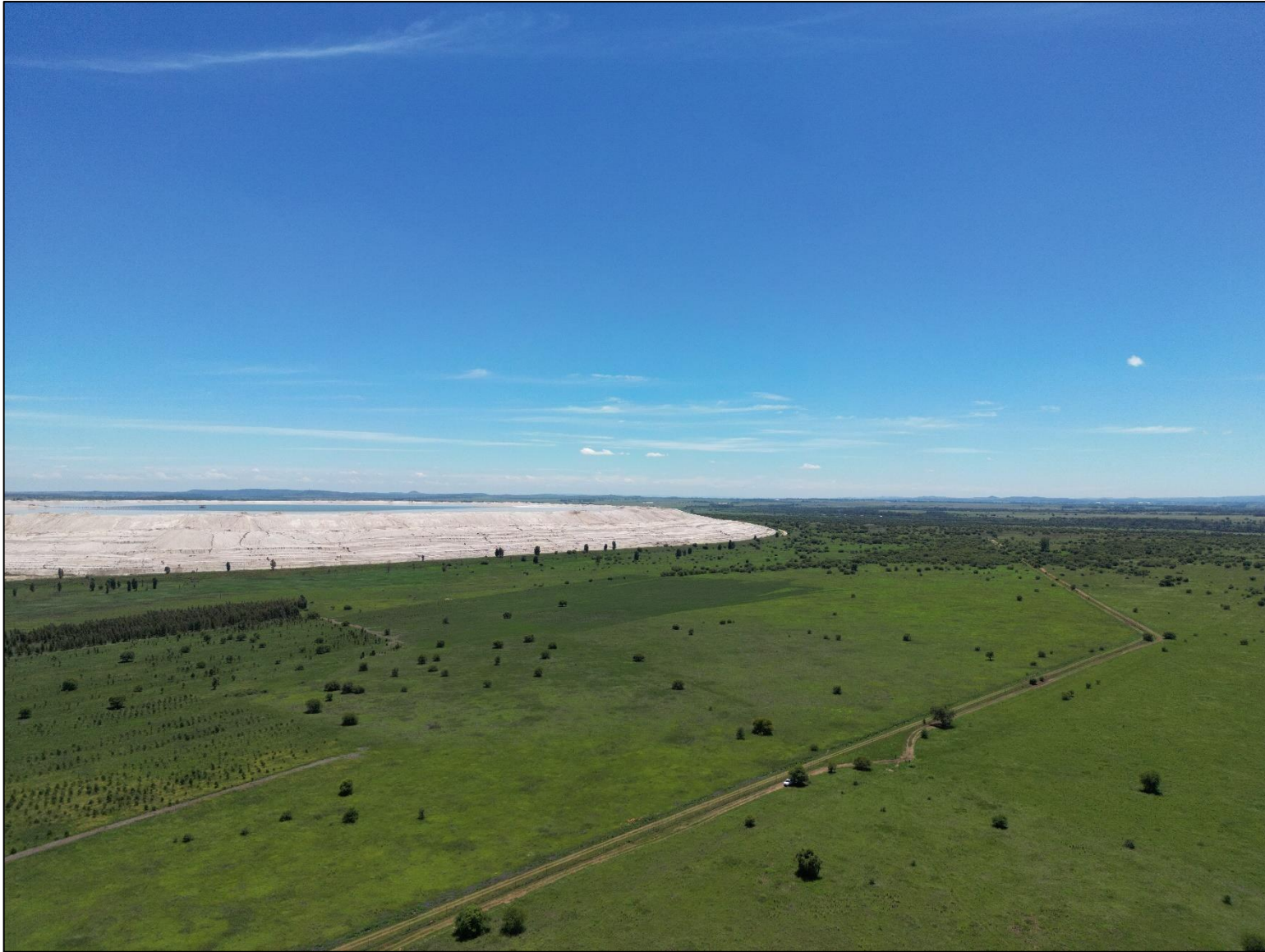
Figure 3.3: Aerial photo at Kareerand BESS taken towards the north-east: AGL 100m
