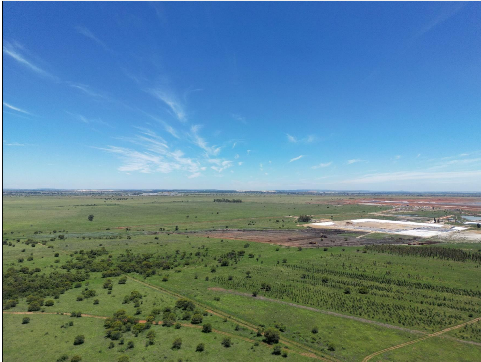
Figure 3.9: Aerial photo at Kareerand BESS taken towards the north-west: AGL 100m
