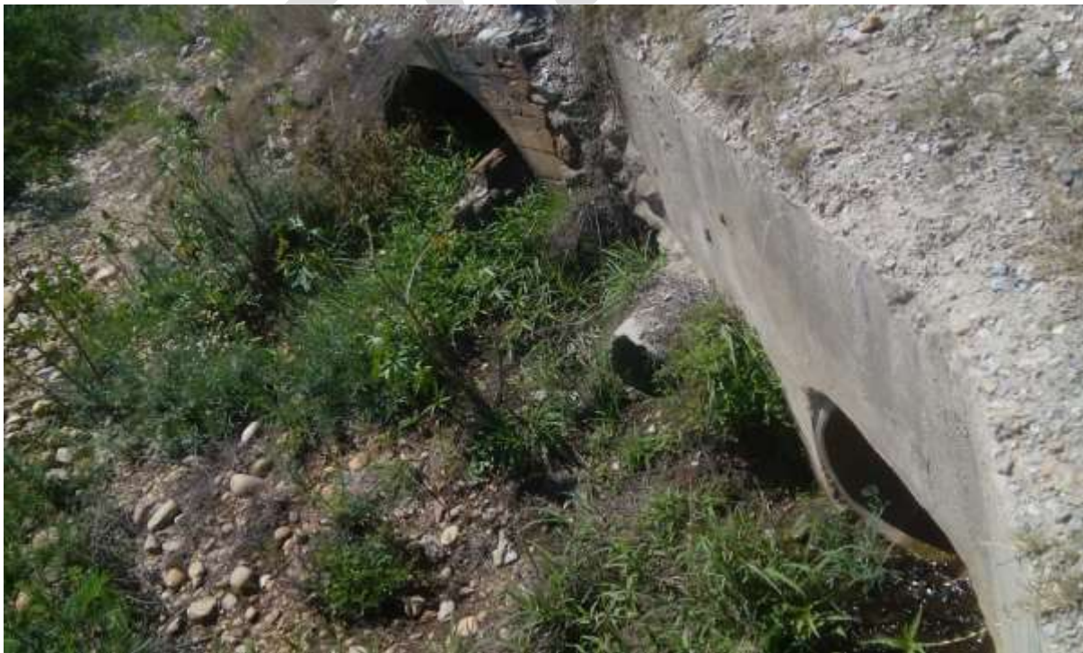
Figure 13: Showing culvert (1x Armco and 2 x concrete pipes) that blocked and caused flooding of adjacent land on GGR.
