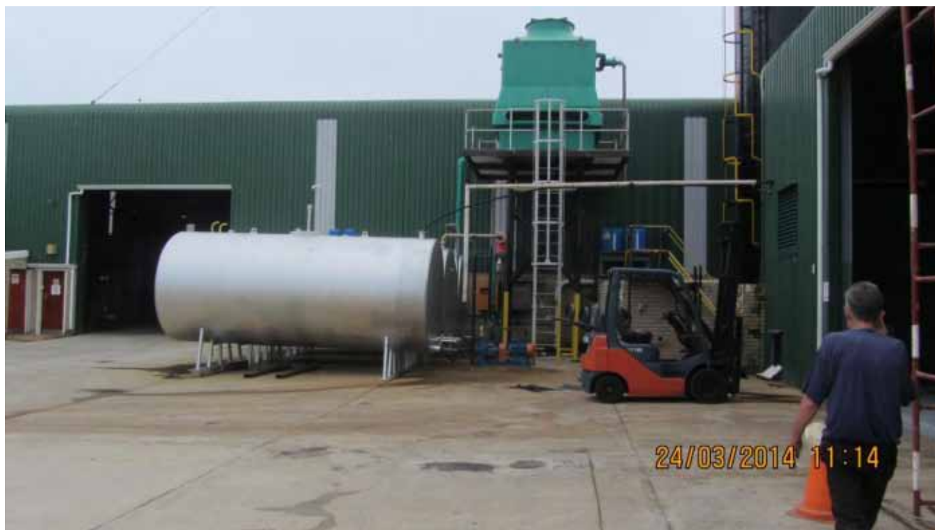
Photo 9: Water cooling tower and recycling system
