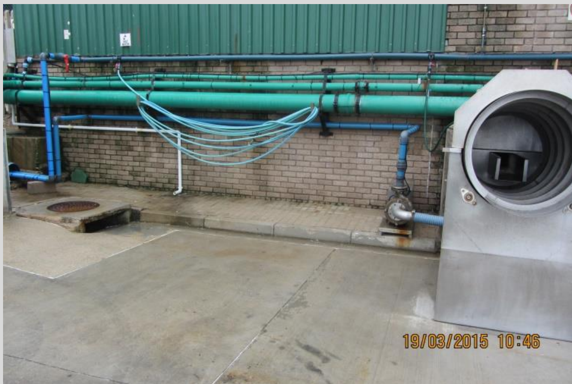
Photo 8: UPVC pipes from the screen running along the wall of the facility
