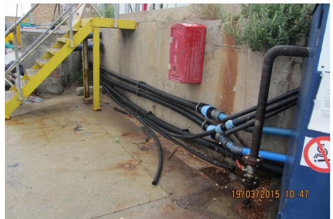
Photo 2: HDPE pipe attached to quay walls
