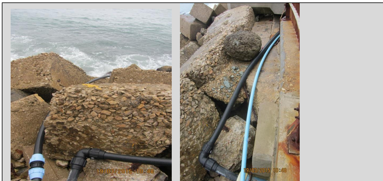
Photo 10: HDPE pipes at the discharge point. Note incoming abstraction pipe.
