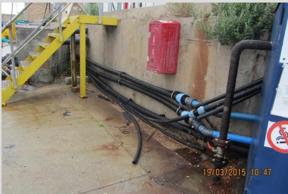
Photo 9: HDPE pipes along the quay to the discharge point
