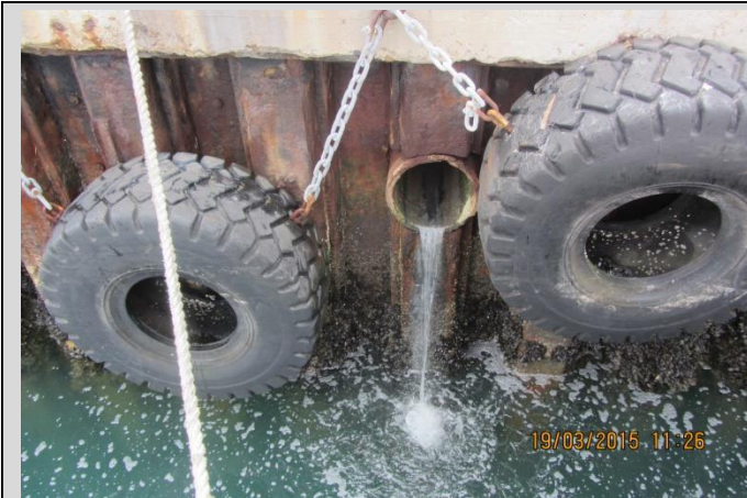
Photo 3: Sea water and ice make up the most of the discharge into the harbour
